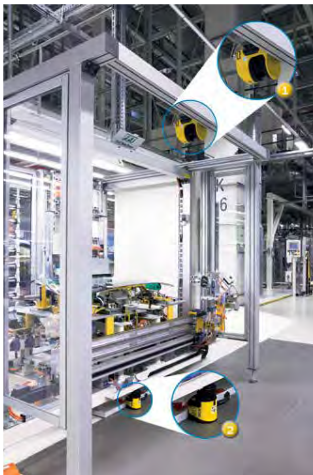
Safety laser scanner on a machine as safety function position 1, initiating a stop and safety function position 2, preventing unexpected start
