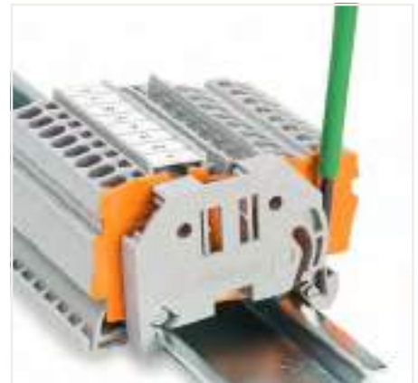
Removing an end stop from the DIN-rail.
