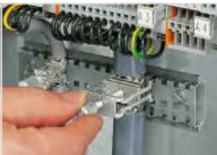
Tightening/removing a shield clamping saddle.
