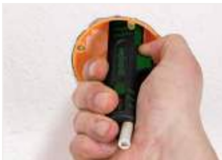
Stripping a cable sheath.
