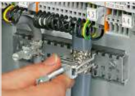
Securing an additional shield clamping saddle.
