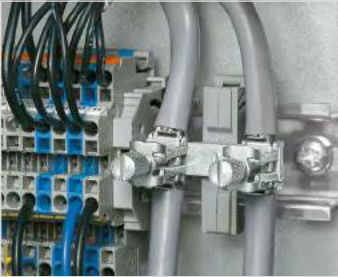
Carrier with grounding foot – busbar parallel to the DIN-rail
