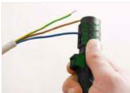
Stripping the conductor insulation.
